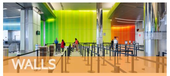
Almost any thickness Lightblocks can be used for wall panels. Thin material can be direct glued to your drywall and thicker materials can be adhered to MDF and hung on zclips. Both materials are offered in fire rated and non fire rated options. In the image, you can see our Class B wall panels on mdf hung on zclips.
